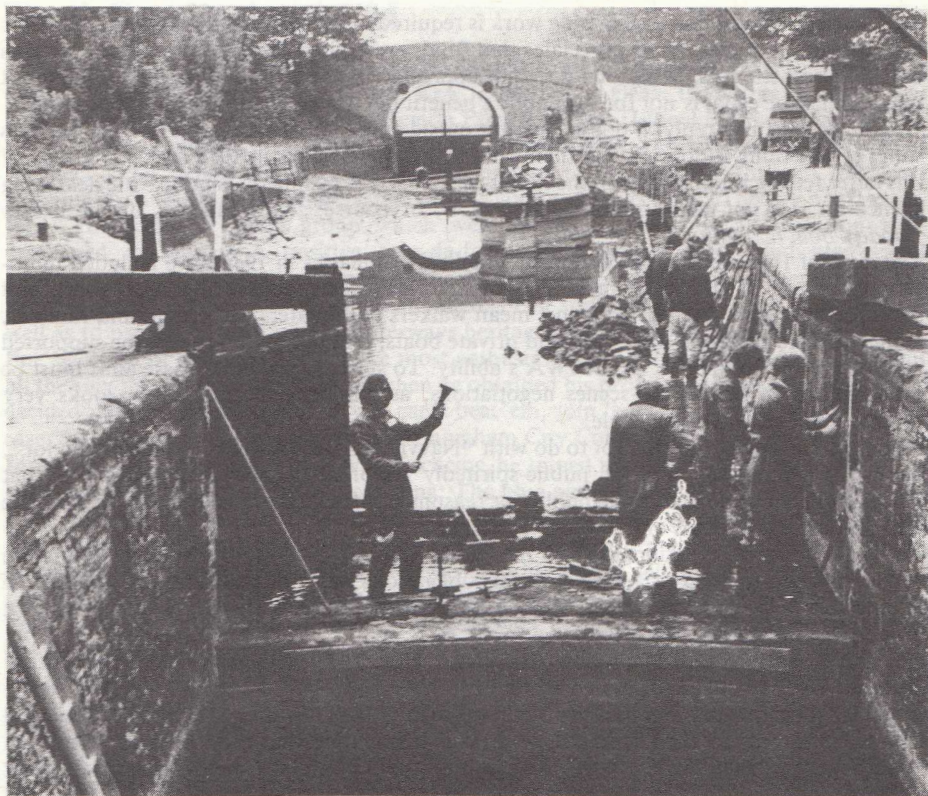
A typical "Out-of-Season" stoppage at Cowley on the GU from 21 October to 11 November, 1979 where three weeks were "needed" to renovate the lock chamber and pile the towpath bank. What price David Hutchings' record of six weeks to build a lock, including approach channels, from 'scratch' in an open field on the Upper Avon?!!
